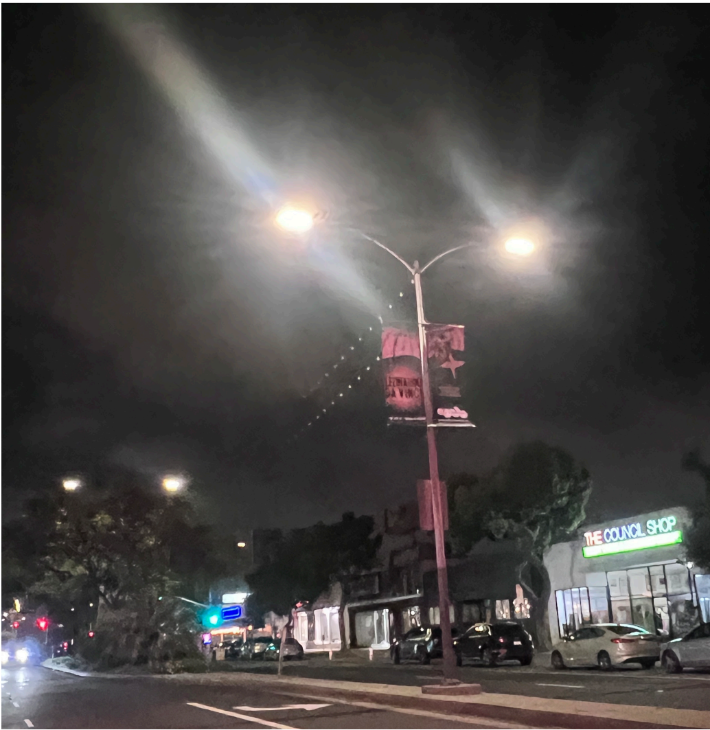
All lights here on Venice at Grandview are broken and non-working.
